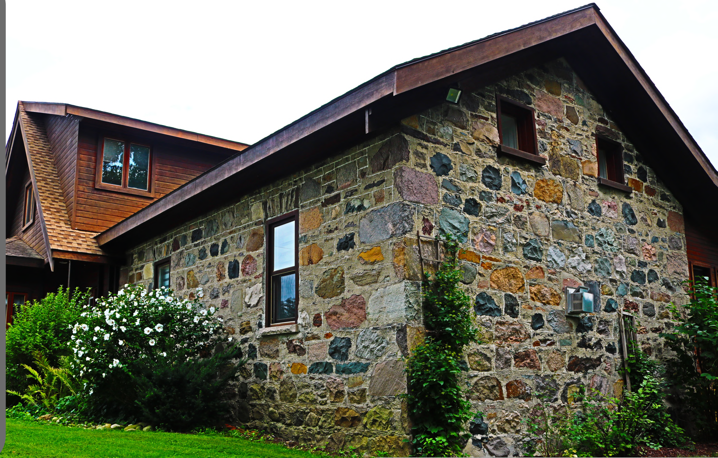
2022 west & north elevation
