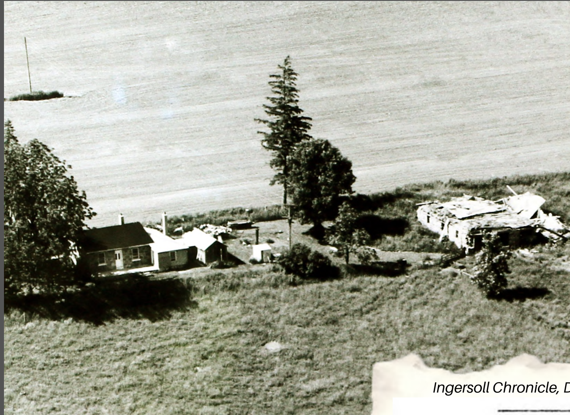
1963 south elevation, photograph from the collection of the Harrison family
